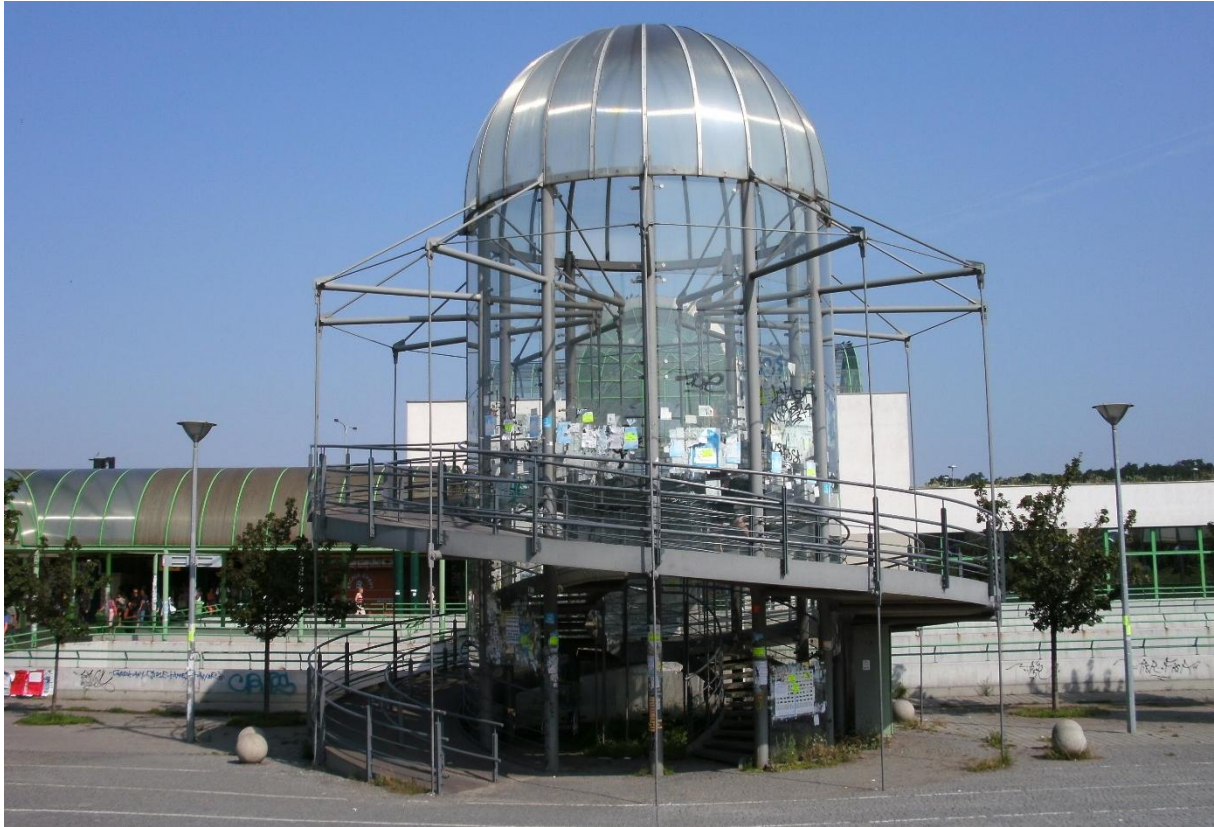
Fig. 3 Example poorly designed barrier-free ramp does not allow independent use (slope and shape) - Prague-Černý Most, (author: Alžběta Bílková, 2013).
